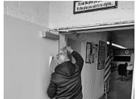
Post 62 New front door being installed and adjusted (photo on March 13, 2024)
