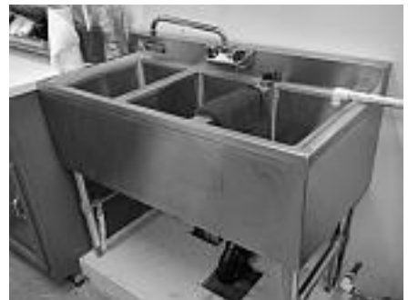
New Sink Installation Done
